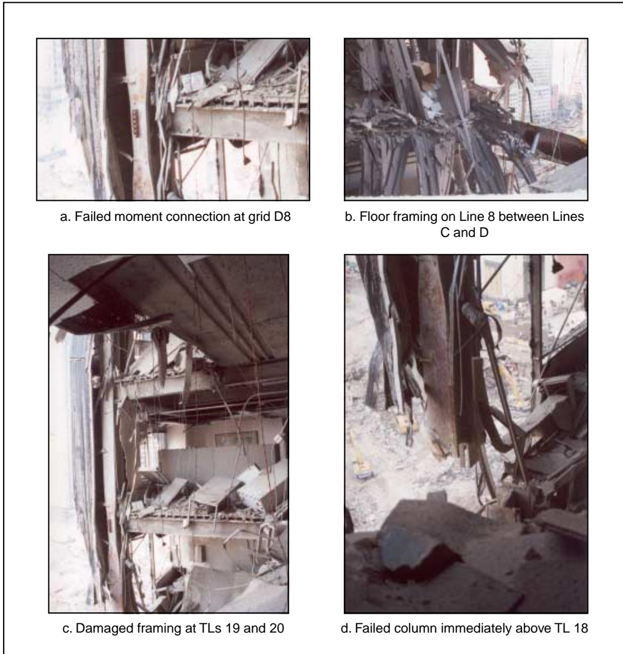
*Figure 2.7. Interior damage photographs from TL 19*
