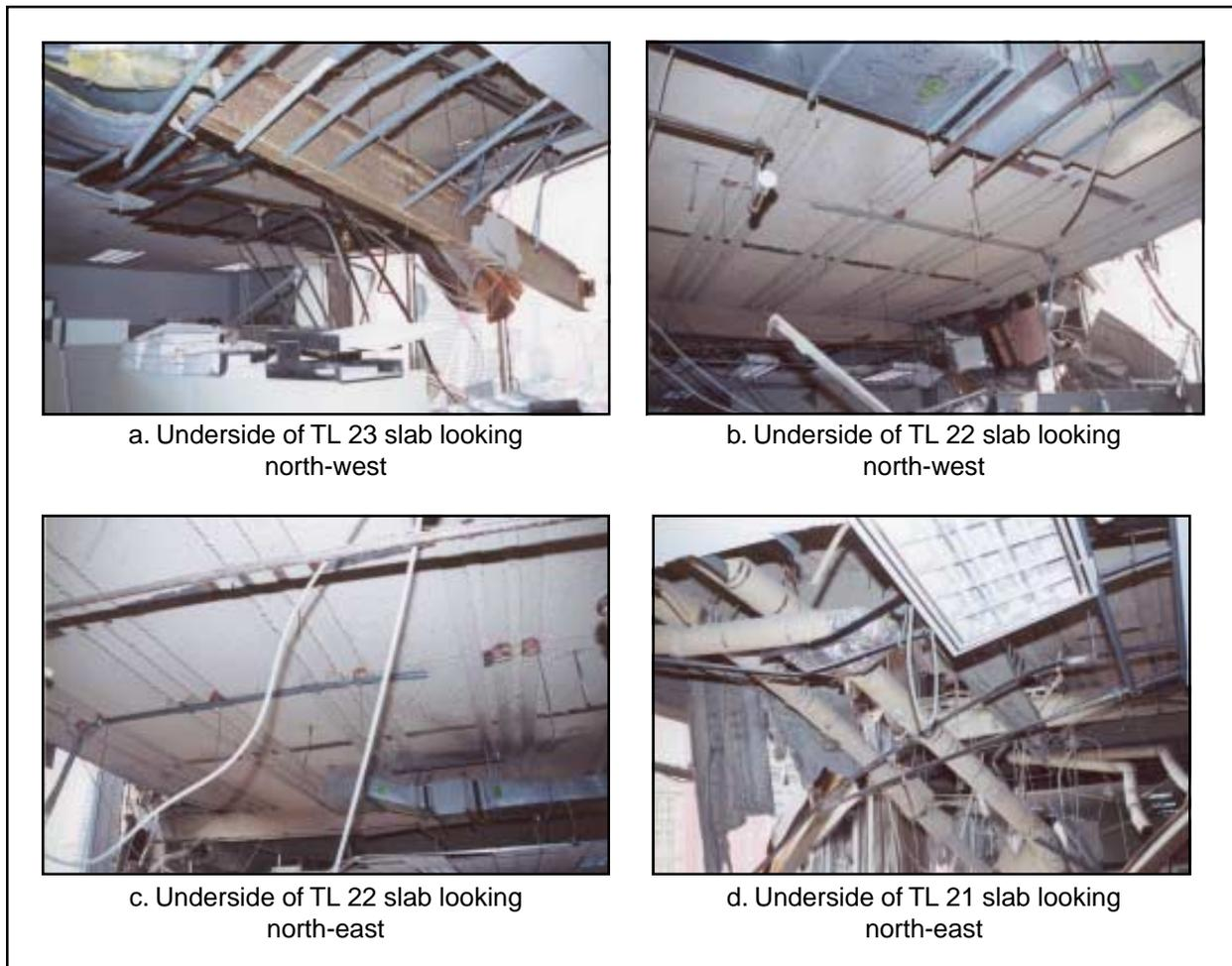
*Figure 2.6. Interior damage at TLs 22 and 21*
