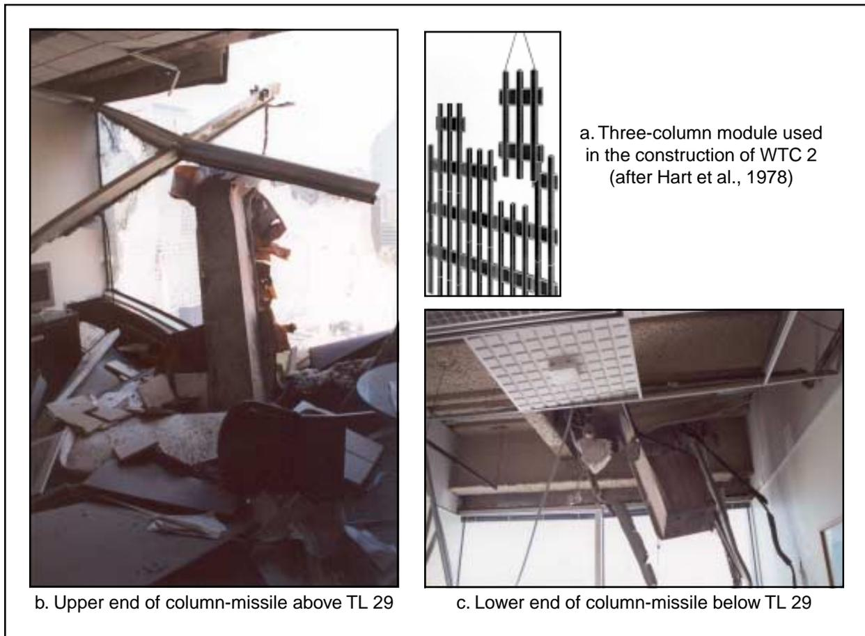
*Figure 2.5. Damage due to column-missile ejected from WTC 2*
