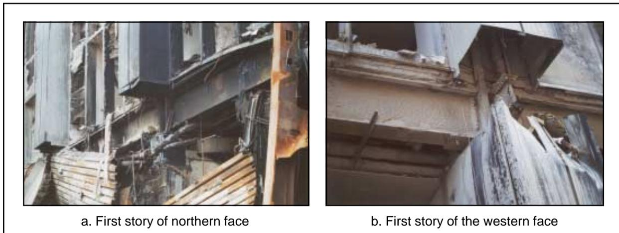
*Figure 2.2. Exposed steel moment framing in the first story of the building*
