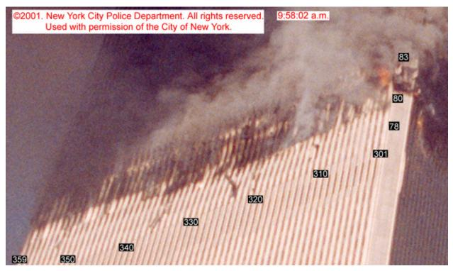
Figure 2–11. Cropped photograph of the east face of WTC 2 at 9:58:02 a.m. The intensity levels have been adjusted, and column and floor numbers have been added.
