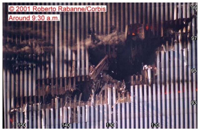
Figure 2–2. Photograph of the north face of WTC 1 around 9:30 a.m. showing the area damaged by the aircraft strike.
