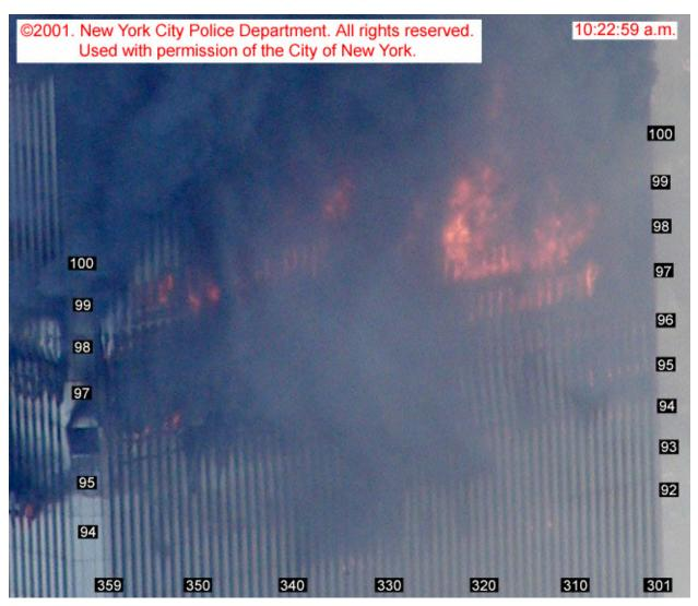
Figure 2–3. View of the south face of WTC 1, cropped from a photograph shot from a helicopter at 10:22:59 a.m. It has been enhanced by adjusting the intensity levels, and column and floor numbers have been added.
