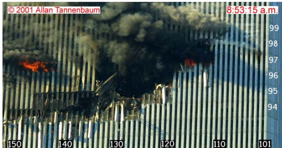
Figure 3–14. Photograph of the north face of WTC 1 recorded at 8:53:15 a.m. on September 11, 2001. Labels showing floor and column numbers were added to the original photograph.
