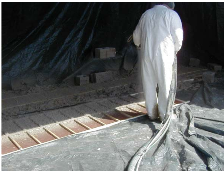
Figure 7–5. Spraying steel plates with BLAZE-SHIELD DC/F.
