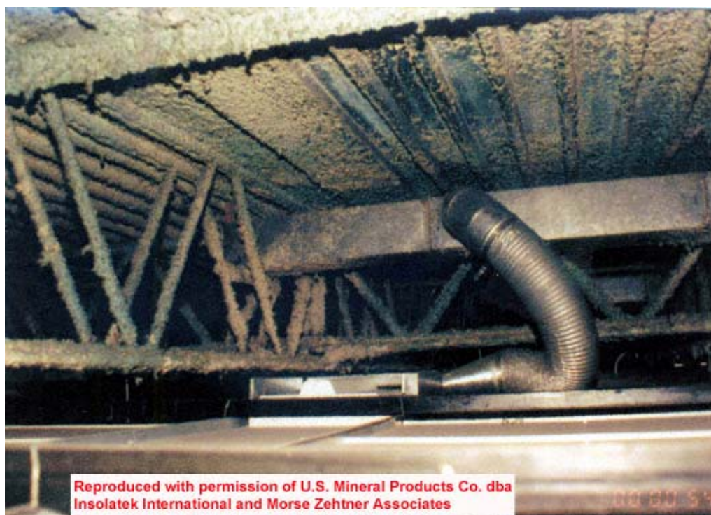
Figure 3–9. Intersection of main truss and bridging truss showing thin SFRM on the ends of some web bars; SFRM was not applied to the metal decking.
