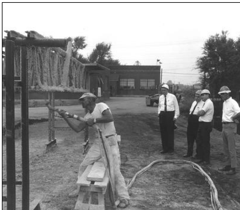
Figure 3–3. Demonstration of application of Monokote sprayed fire-resistive material to floor trusses.
