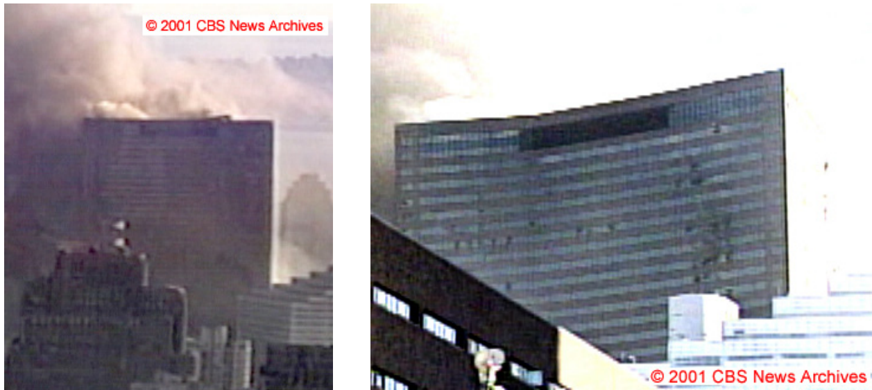
Figure 5–203. Cropped frames from the Camera 2 video clip in Figure 5–185 and the Camera 3 video clip in Figure 5–186, showing the north face of WTC 7 9.0 \text{ s} \pm 0.1 \text{ s} after the east penthouse began to move downward. The intensities have been adjusted.
