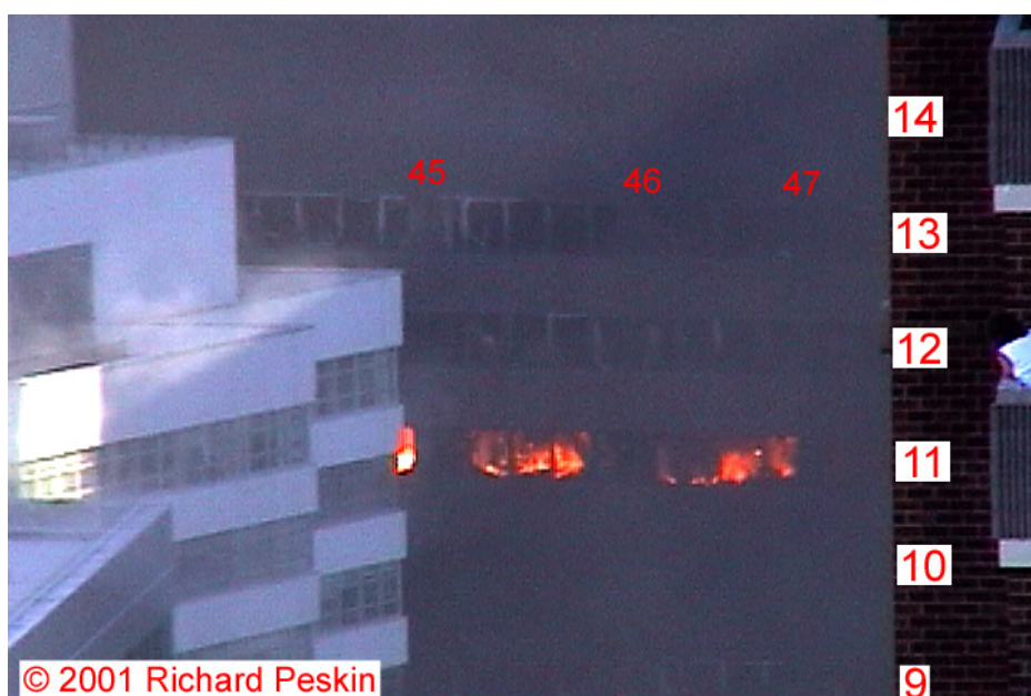
Figure 5-149. Frame from a video clip showing a close up view of the north face of WTC 7 at 4:38:14 p.m. \pm 1 s. The video was shot from the same location as the frame in Figure 5-147. The image intensities were adjusted, and column and floor number have been added.
