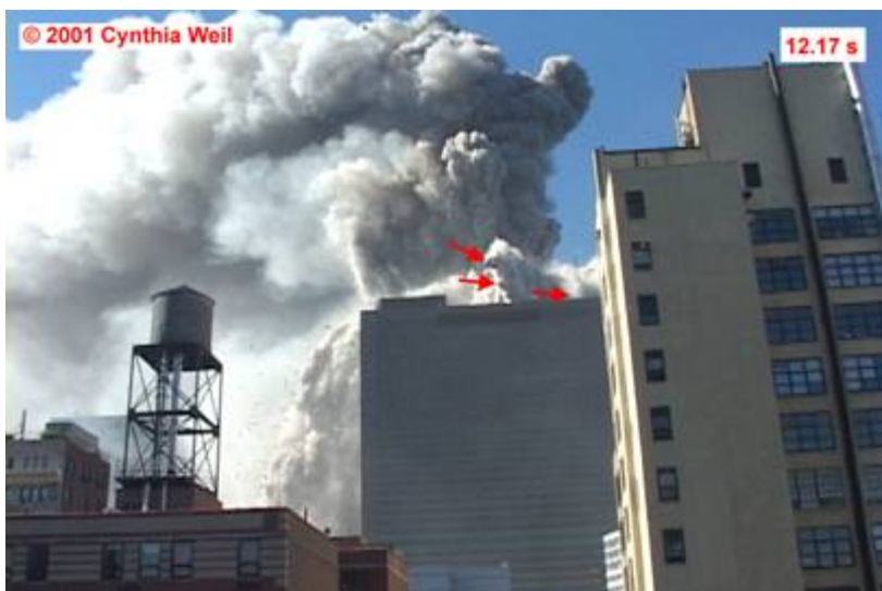
Figure 5–41. Three pairs of frames taken from videos shot from the north and west, showing the collapse of WTC 1. Times are relative to the start of the collapse. Arrows indicate large objects that were projected toward WTC 7. The intensities of the video frames have been adjusted.
