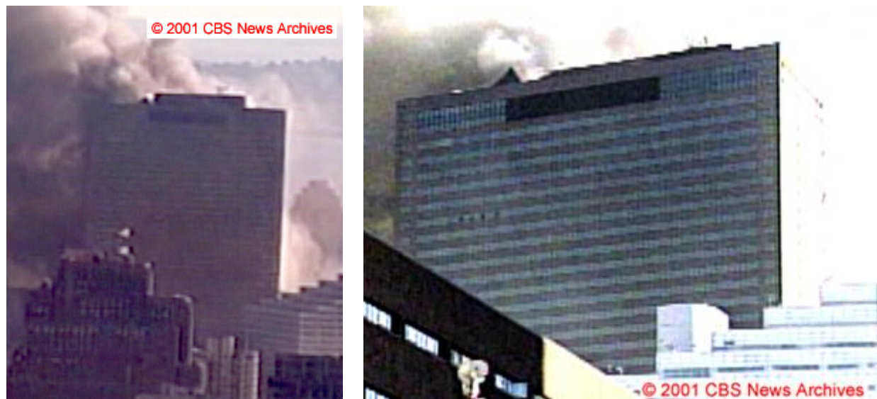
Figure 5–195. Cropped frames from the Camera 2 video clip and the Camera 3 video clip, showing the north face of WTC 7 1.7 \text{ s} \pm 0.1 \text{ s} after the east penthouse began to move downward. The intensities have been adjusted.
