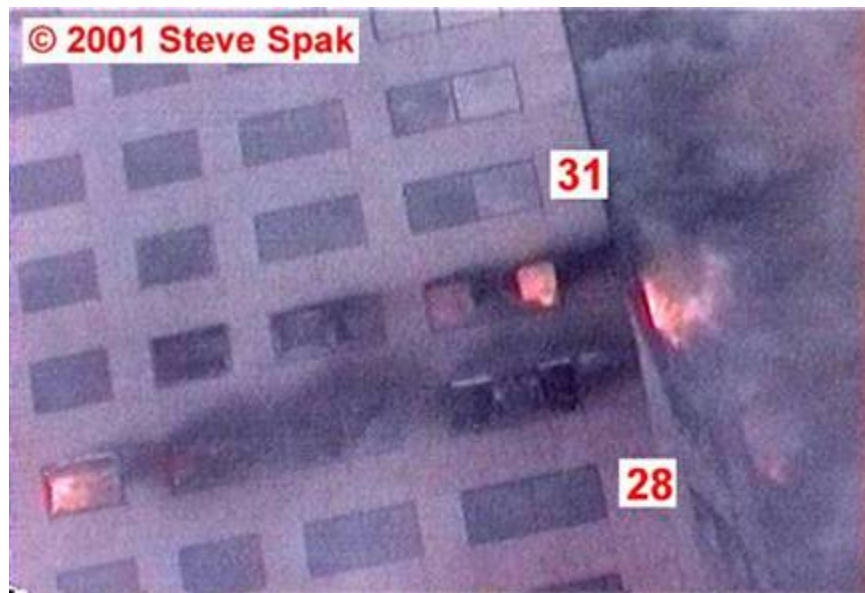
Figure 5–111. Frame from a video clip showing fires near the southwest corner of WTC 7 on the 29 th and 30 th floors around 12:28 a.m. ± 3 min.
