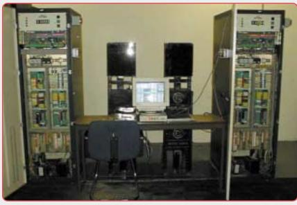
Elevator machine room showing typical installation of SWIFT controller
